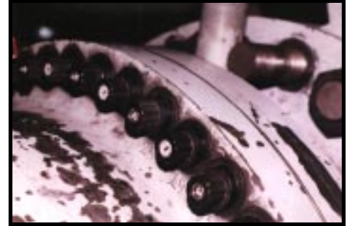
Load indicating fasteners assure the integrity of this flange for a large blast thermal simulator that carries gas under high pressure sufficient to simulate a nuclear explosion shock wave when released.
